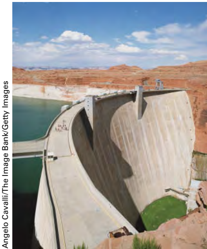
Glen Canyon Dam at Lake Powell, Arizona
