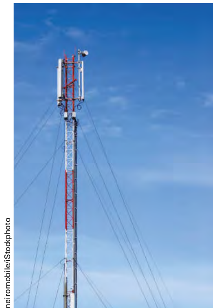
The three-dimensional equilibrium of the cell-phone tower must be carefully analyzed so that excessive net horizontal force applied by the cable system is avoided.
