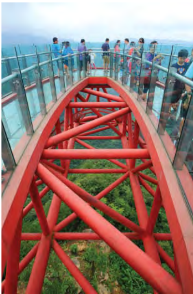
A space truss is incorporated into the world's longest glass skywalk which is located in Huangshi National Forest Park in Chongqing, China.
