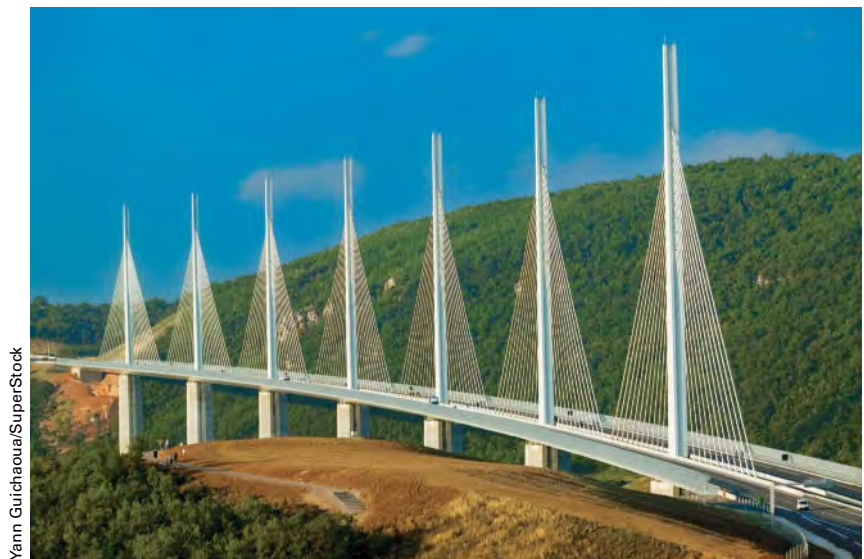
The Millau Viaduct in southern France. Note that the full height of the pylons is obscured here.
