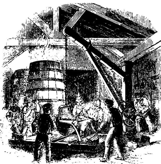
107 Nineteenth century stove cupola
