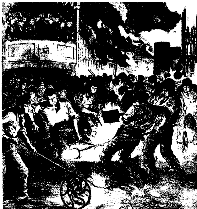
139 The Prince of Wales watches the pouring of an ingot of crucible steel in the Norfolk Works of Thos. Firth and Sons in 1875; the weight of the ingot cast was probably no more than 20 t (courtesy of Firth Brown Ltd, Sheffield)
